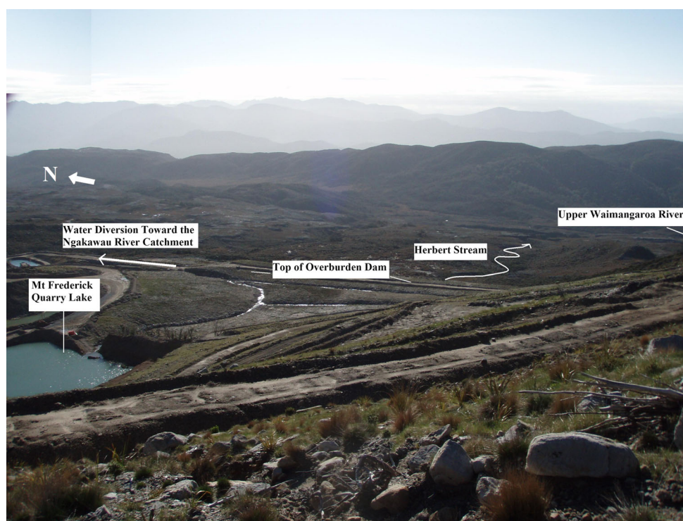
Fig. 2 The study area looking east from Mt Frederick. Water from above the overburden dam is diverted north to avoid contamination of the Waimangaroa River, but Herbert Stream, which rises from leakage of the overburden dam, is AMD affected
